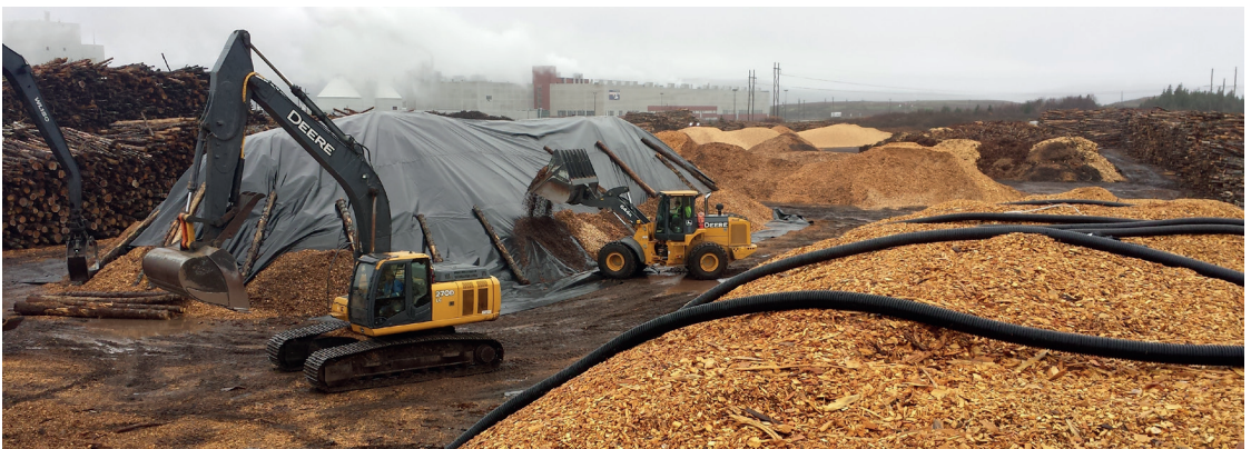
Figure 10. Recommended storage practices for fuel chips.
