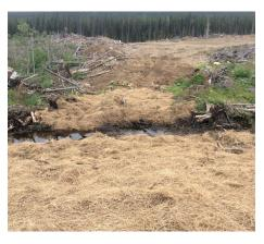
Access management Deactivated roads should be barricaded to prevent access by motor vehicles other than ATVs. Berms built from local earth and rock are the preferred form of barricade. All access berms must be clearly marked and visible to all traffic.
