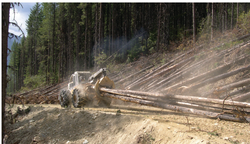
Figure 4. Skidding on the finished road grade was one variation in the construction technique used at the SP5 Road location.
