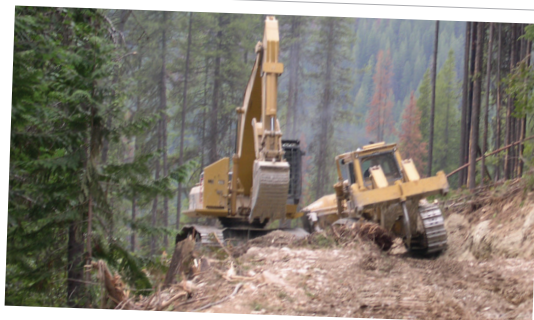
An excavator and a crawler-tractor were used for roadbed and landing construction.
