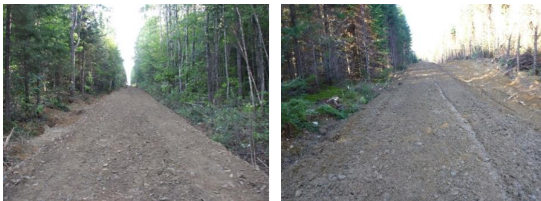
Figure 3. Final road surface, as completed by the Kobelco BladeRunner ED150 (left) and the excavator and bulldozer team (right).
