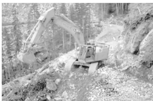
Figure 4. Excavator ripping rock with bucket.
