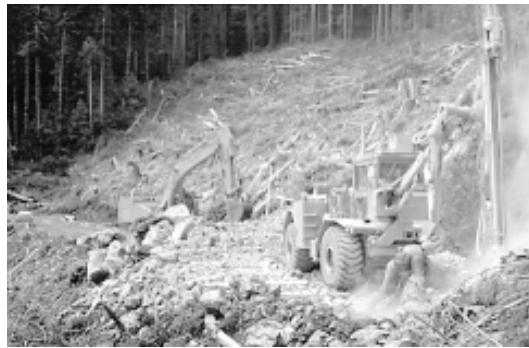
Figure 5. Rockdrill at work while excavator loads truck.
