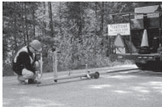
Figure 4. Taking Benkelman beam measurements.
