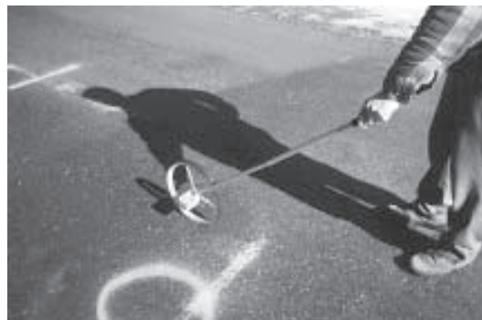
Figure 5. Measuring crack length in a surface distress survey.
