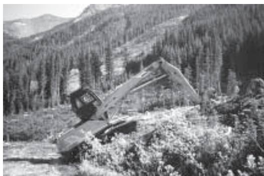
Figure 3. Loader entering Cutblock 21 at a location with low cutbank height.
