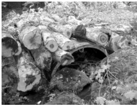
Figure 2. Corduroy helps to protect the arch and to distribute the load imposed by passing equipment.
