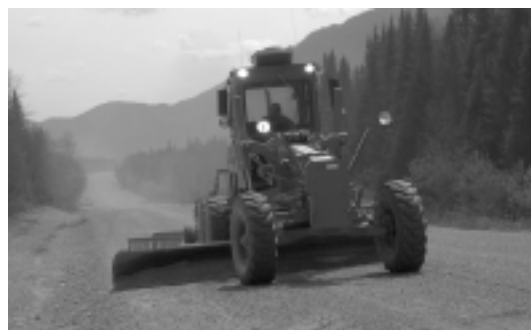
Figure 1. Grading a forestry road.
