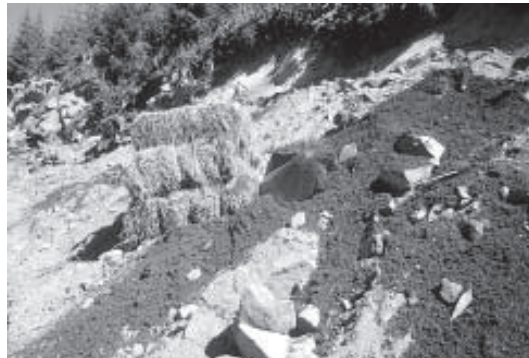
Figure 5. Compost mixed with pulled-back sidecast.
