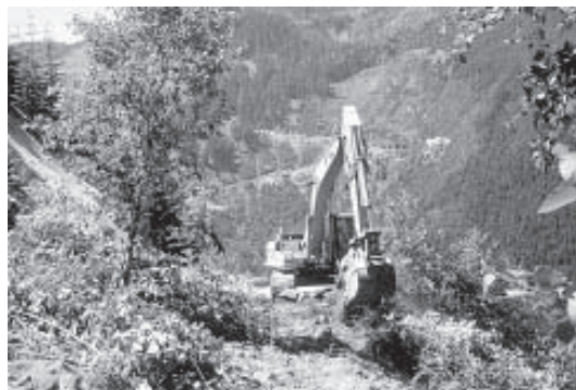
Figure 6. Excavator restoring original slope to deactivated logging road.
