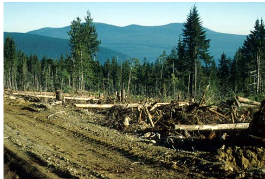
Figure 5. Decking area prepared by a loader-forwarder.
