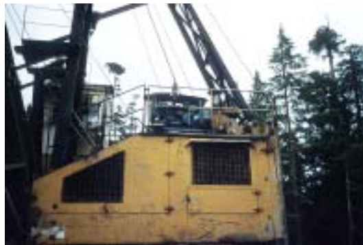
Figure 2. Light plant mounted on the deck of the yarder house.
