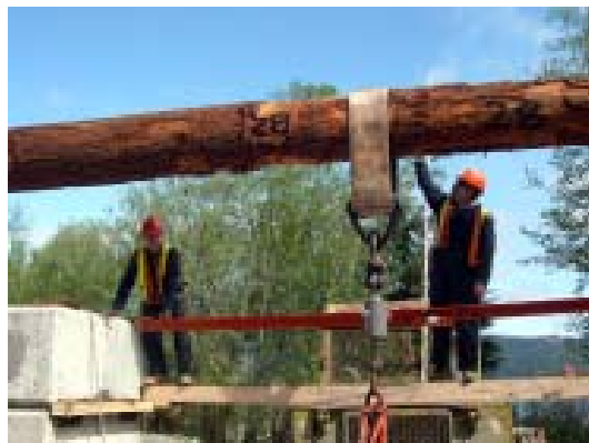
Figure 6. Connecting transducer draw-wire to log.
