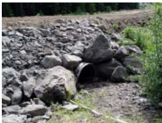
Figure 12. Inlet of arch showing placement of large and small riprap on fill slopes around the arch.
