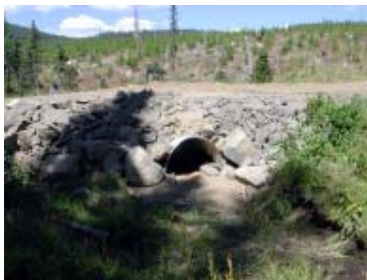
Figure 13. Outlet of arch at Esperon Road site showing fill height above arch and the low areas on either side of the arch along the road.
