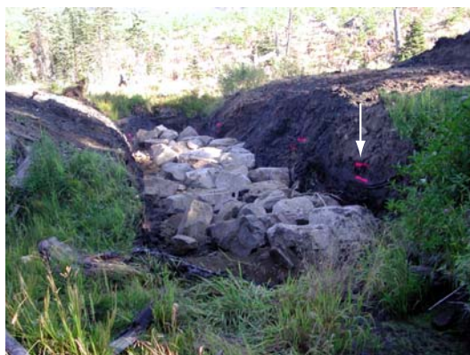
Figure 8. The Esperon Road site showing first lift of large riprap before topping with crushed aggregate. Arrow indicates design height of fill.
