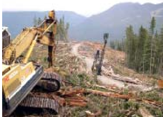
Figure 2. Cypress 7280 yarder and mobile backspur working in the upper (southern) part of the block.
