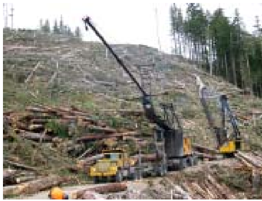
Figure 3. Cypress 6280 yarder and line loader working in the lower (northern) side of the block.
