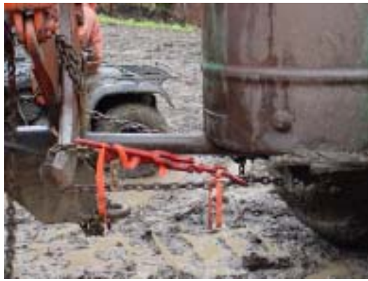
Figure 5. Example of temporary tank attachment method.
