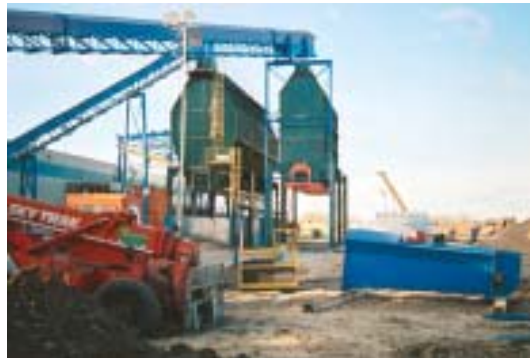
Figure 3. Overhead bins for pulp chips (left) and hog fuel (right).
