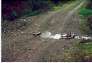
Figure 62. Photo and schematic of typical waterbar.
