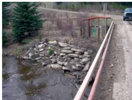
Figure 77. Used concrete keyed together to armour against stream bank erosion below a bridge abutment.
