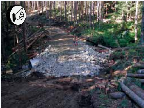
Figure 35. New road construction showing aggregate placed along the approaches and embankments of a fish-stream crossing (embedded culvert).
