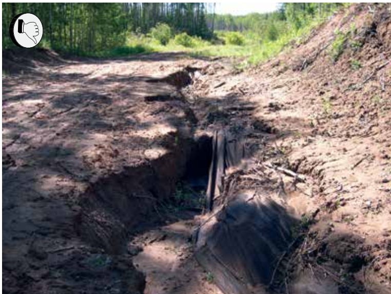
Figure 48. Ditch showing signs of downcutting and poorly functioning geotextile.
