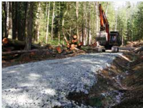
Figure 33. Crushed aggregate placed along a newly built road.
