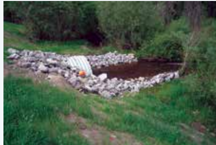
Figure 78. Before-and-after photos of an embankment above a culvert showing the use of a fibrous mat and reclamation seed mix (photo courtesy of Hinton Wood Products – a division of West Fraser Mills Ltd.).
