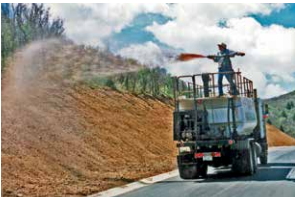
Figure 20. Hydromulching from roadside with a truck-mounted unit (photo courtesy Canadian Forest Products Ltd.)
