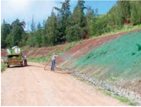
Figure 21. Hydroseeding with a trailer-mounted unit using a delivery hose. The hose allows the forest worker to work on or off the road and away from the trailer during application (photo courtesy Canadian Forest Products Ltd.).
