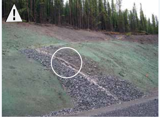
Figure 45. Same diversion channel as Figure 44 after a rainfall event showing water flowing down and through the aggregate apron.
