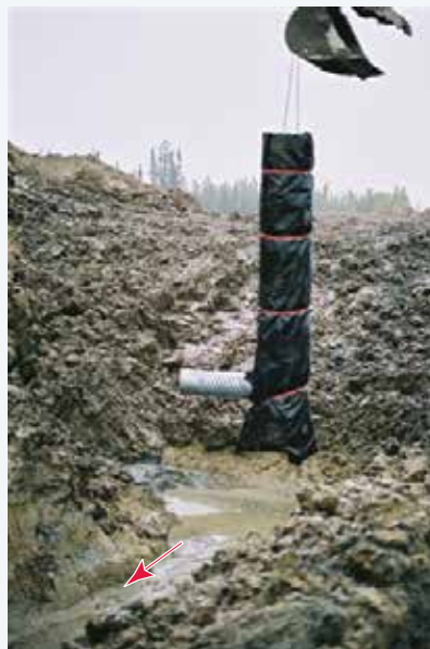
Figure 108. (above) A stand pipe with protruding elbow is wrapped with geotextile and placed directly over a seepage site amongst an outcrop of heavy clay during road construction. (left) The prepared perforations along the inside of the pipe (photo courtesy of Millar Western Forest Products Ltd.).
