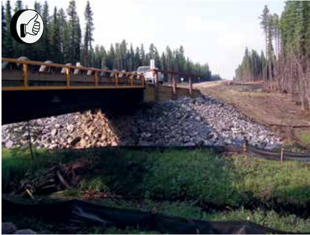
Figure 16. Undisturbed riparian vegetation below recently installed bridge. Note the use of aggregate and a geotextile fence for erosion and sediment control.
