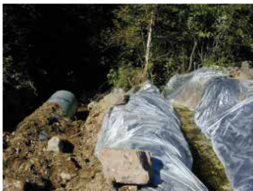
Figure 88. An open trench diversion is used to dewater a stream channel. The plastic lining will prevent erosion of the trench itself.
