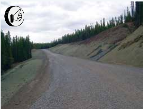
Figure 10. Same section of road as Figure 9 after second application of surfacing aggregate to further reduce erosion hazard and prepare surface for more traffic.
