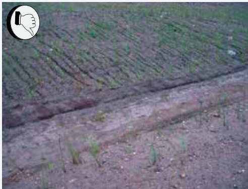
Figure 3. Rills formed along a fillslope showing orientation predominantly straight downslope.
