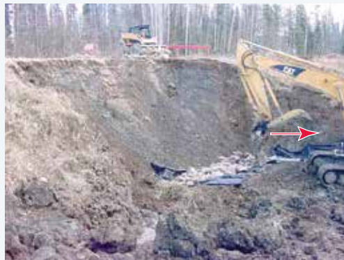
Figure 106. Same site as Figure 104 showing the construction of a subsurface drain made of aggregate wrapped with a geotextile.
