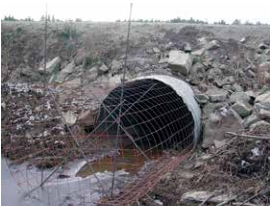
Figure 92. An extension attached to the inlet of a culvert is intended to prevent blockage of stream flow due to beaver activity.
