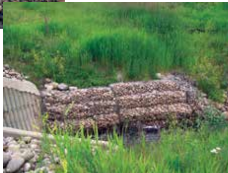
Figure 76. Wire-mesh gabions filled with aggregate used to armour a stream bank at the inlet of a culvert.
