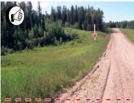
Figure 79. A ditch is turned out (see arrow) where the surrounding terrain allowed, rather than uphill from this location where the terrain would not accommodate it. The dashed line indicates a culvert position.
