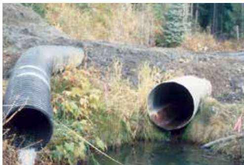
Figure 86. Outlet of a large diameter diversion pipe (left) showing stream flow re-entering the channel during preparation for the replacement of the perched culvert (right).
