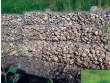
Figure 75. Smaller aggregate placed inside wire-mesh gabions.
