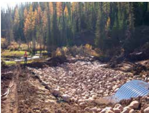
Figure 73. Inlet of culvert showing a section of newly constructed stream channel armoured with aggregate. The construction site is dewatered and the stream flow has not been re-introduced to the new channel.
