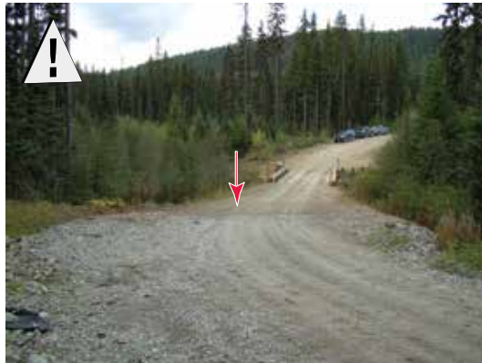
Figure 103. Where older existing bridge decks are located at a low elevation along the road alignment, water interception techniques should be used to divert road surface flows from reaching the deck and entering the stream. The arrow indicates the position of the open-top surface drain seen in Figure 64.
