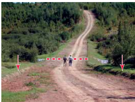
Figure 68. Roadside berms (see arrows) used to contain water and sediment on the road surface to protect and minimize sediment delivery to a watercourse crossing (see dashed line). A controlled breach of the berm is located away from the watercourse crossing.
