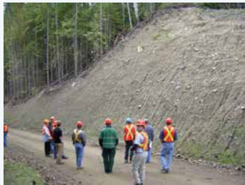
Figure 19. Steep continuous slope showing poor germination after dry-seeding.
