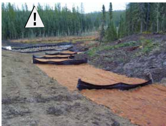
Figure 81. Fibrous matting is used to armour a turned-out ditch against erosion, and geotextile fences were built to promote deposition of sediment. The maintenance required for the fences (removal of deposited sediment) may damage the fibrous matting.
