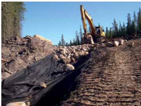
Figure 81. Fibrous matting is used to armour a turned-out ditch against erosion, and geotextile fences were built to promote deposition of sediment. The maintenance required for the fences (removal of deposited sediment) may damage the fibrous matting.
