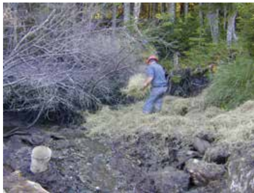
Figure 30. Forest worker spreading straw over exposed soil as an erosion control measure.
