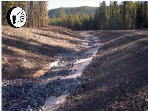
Figure 49. New road construction showing ditch lined with fibrous matting and aggregate.
