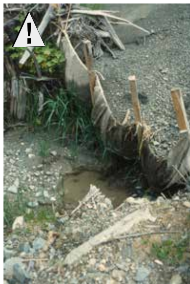
Figure 38. Fence made from burlap and wooden stakes showing deposition of material on the uphill side.
