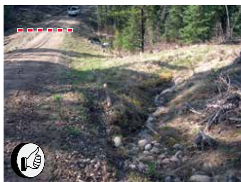
Figure 56. The photo shows a ditch that has been turned to direct flows into the forest, which prevents direct delivery of sediment to the stream at the bottom of the slope (see dashed line). The schematic shows a ditch turned into the forest with aggregate placed in the flow path to prevent erosion and to promote deposition of sediment.
