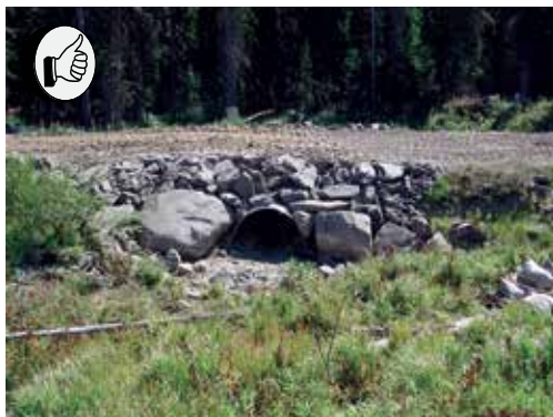
Figure 71. Aggregate armouring placed around the inlet of an arch culvert. The larger sized material is placed to direct high flows through the culvert and protect against scour, whereas the smaller sized material is placed further upslope mainly to control erosion.
