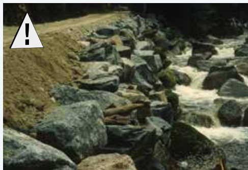
Figure 13. Aggressive aggregate armouring of older road adjacent to river with no riparian area remaining.
