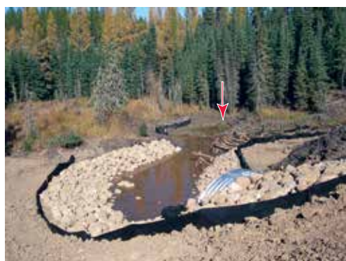
Figure 74. Outlet of newly installed culvert showing aggressively armoured stream bank and a geotextile fence to prevent sediment from migrating towards the stream. The arrow indicates rot-wad structures installed for aquatic habitat diversity.
