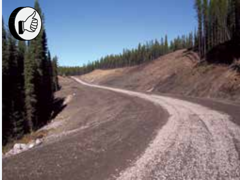
Figure 9. Newly built road with initial surfacing aggregate to satisfy immediate erosion hazards during construction.
