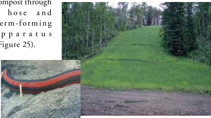
Figure 23. Compost “socks” (see inset) are easily prepared and positioned on-site (photos courtesy of Top Spray, a division of Spray Lake Sawmills [1980] Ltd.).
