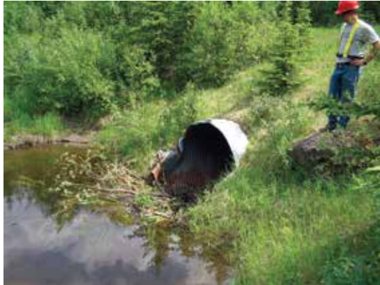
Figure 91. Recent beaver activity at the inlet of a culvert (photo courtesy of Hinton Wood Products – a division of West Fraser Mills Ltd.).
