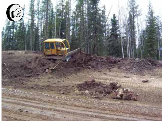
Figure 31. Crawler-tractor spreading logging debris and reclaimed topsoil over an exposed slope.
