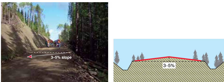
Figure 66. The photo shows an insloped road, built to direct flows towards the ditch (see direction of arrow) and away from the fillslope. The schematic shows a general view of a crowned road surface.
