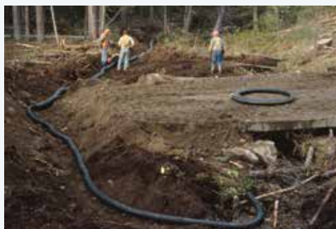
Figure 85. Preparing to divert stream flow through a flexible pipe during the replacement of a temporary concrete slab crossing.
