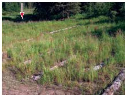
Figure 70. Non-merchantable logs placed parallel to each other across the contour create a terracing effect to capture sediment. The slope was successfully seeded and riparian vegetation was protected adjacent to the nearby stream (see arrow).
