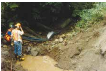
Figure 84. Outlet area along an excavation during a culvert installation showing pumped stream water re-entering the stream. A sump is used to collect sediment-laden seepage and prevent it from leaving the construction site and entering the stream.
