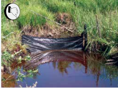
Figure 39. A geotextile fence placed across a slow-flowing channel during a nearby culvert installation.
