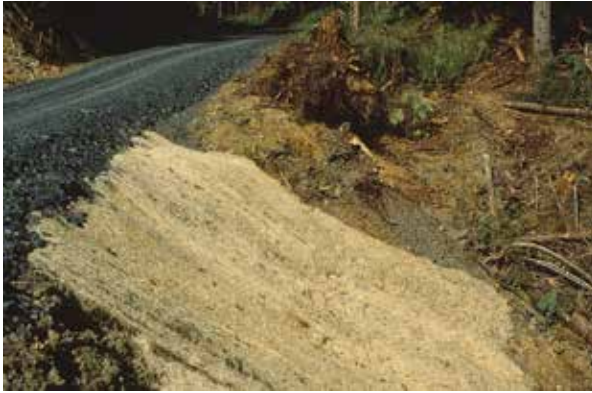
Figure 29. An erosion control blanket placed on a fillslope.
