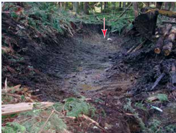
Figure 89. View of seepage along an excavation during the installation of a culvert and a prepared sump at the outlet (see arrow).
