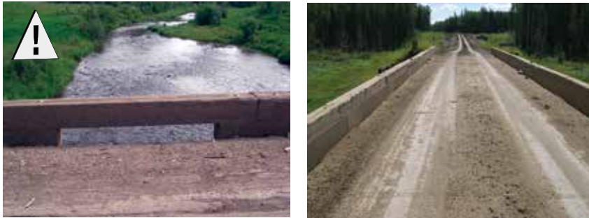
Figure 95. Two bridges with similar guardrails, but one has been left open while the other has been retrofitted with steel plates to block the openings and prevent the deposit of sediment into the stream below.
