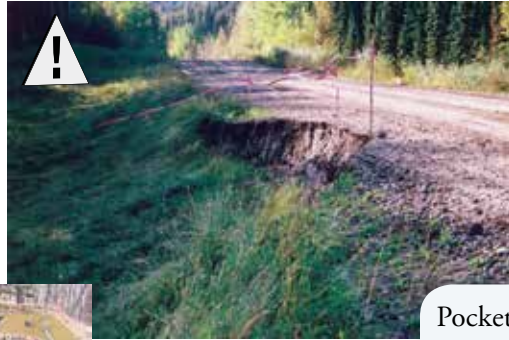
Figure 104. Road edge failure due to saturated soils from seepage and subsurface flows below the road has resulted in sediment delivery towards a nearby stream.
