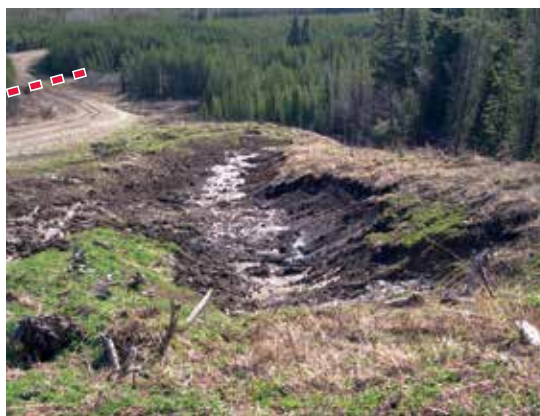
Figure 109. Exit area of French drain showing diversion channel directing water away from the road and into the forest. The dashed line indicates the location of a fish bearing stream.
