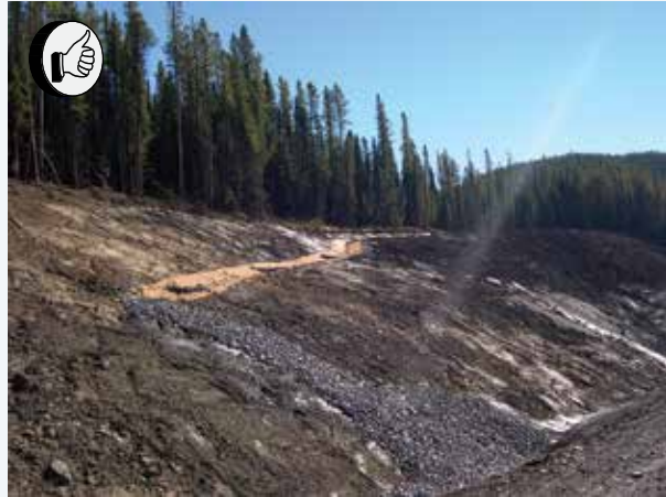
Figure 44. Diversion channel lined with fibrous matting and aggregate check dams.
