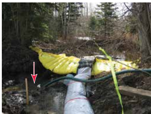
Figure 87. A Water-Gate™ dam and its diverter tunnel were used to direct stream flow around a culvert replacement construction site. A sump was still required (see arrow) to collect seepage flow from in front of the dam, typical with saturated soils below a natural stream channel.
