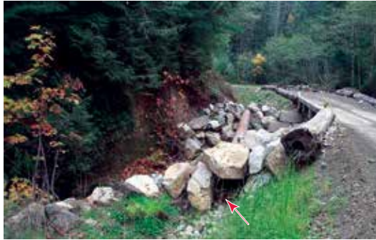
Figure 57. A steel pipe is used to bypass ditch water (see arrow) over a stream (photo courtesy of Island Timberlands Limited Partnership).
