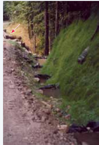
Figure 53. Ditch check structures built from aggregate wrapped with geotextile.
