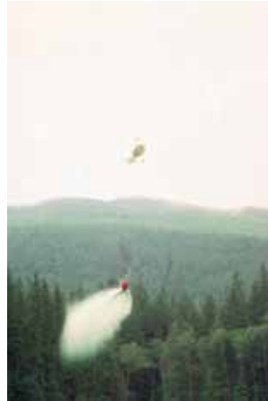
Figure 22. Helicopter hydromulching can treat a large area in a short period of time. In this example, the application rates for the slurry mix were 60 kg/ha of seed mix, 300 kg/ha of slow release fertilizer, 25 kg/ha of tackifier, and 50 kg/ha of mulch.
