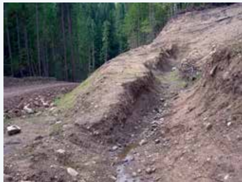
Figure 46. Diversion channel built to address upland seepage flows.
