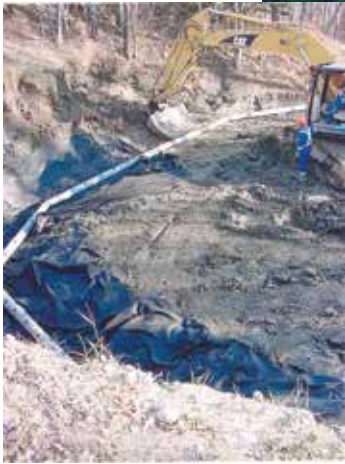
Figure 105. Construction of a subsurface drain made of perforated plastic pipe wrapped with a geotextile.
