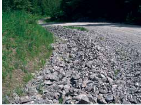
Figure 34. A ditch lined with a continuous blanket of angular aggregate to prevent erosion and control sediment.
