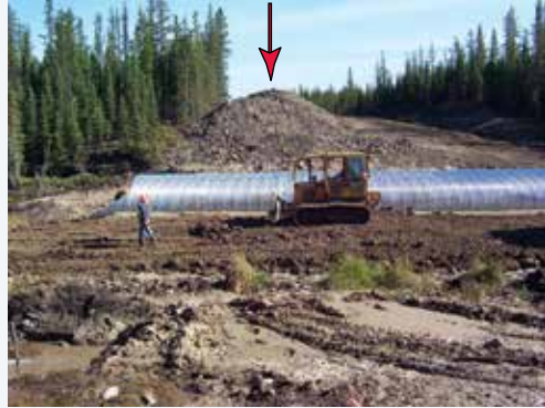
Figure 90. Stockpiled material (see arrow) during a culvert installation.
