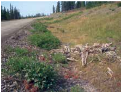
Figure 54. A ditch showing established vegetation and check structure built from logging debris (photo courtesy of Hinton Wood Products – a division of West Fraser Mills Ltd.).
