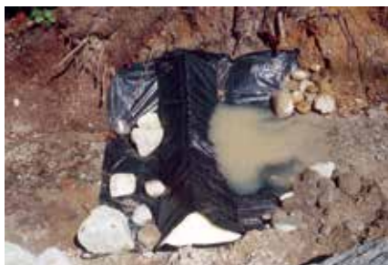
Figure 55. A recently installed ditch check structure using a Triangular Silt Dike™. The foam inside the geotextile wrapping conforms well to irregular surfaces.
