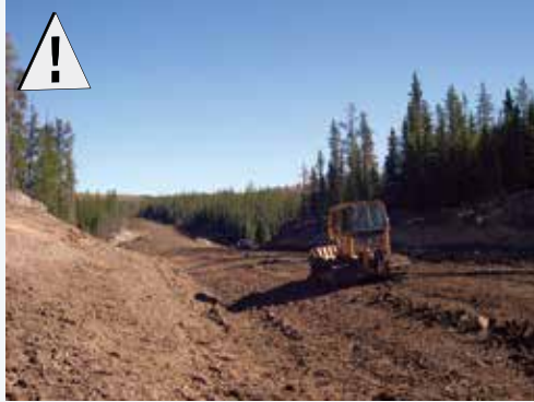
Figure 6. Newly built road showing exposed soil and a cutbank and running surface vulnerable to erosion.
