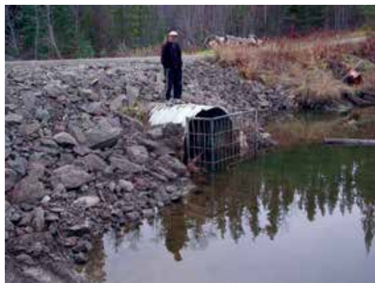
Figure 93. A grate attached to the inlet of a culvert is intended to prevent blockage due to beaver activity.
