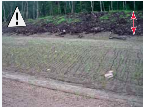
Figure 32. Cutslope showing logging debris and reclaimed topsoil spread over the upper portion and severe rilling along the untreated lower slope.
