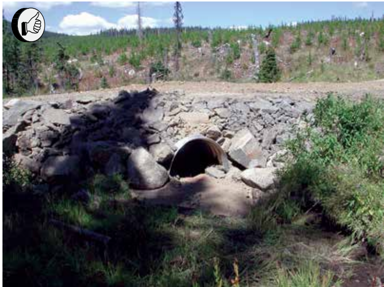
Figure 83. The vertical alignment of the road over the culvert results in the road surface water flowing away from the crossing and stream channel.
