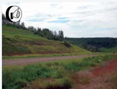
Figure 7. Well covered ditchline and cutslope along older road.
