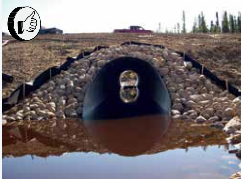
Figure 72. Outlet of 3-m-diameter culvert showing rounded rock used for armouring the fillslope, and a geotextile fence to prevent the migration of sediment towards the stream.
