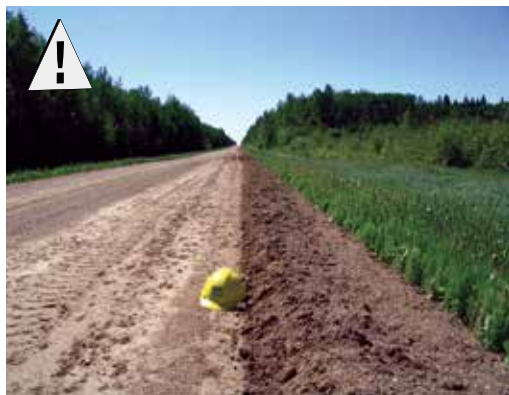
Figure 67. A temporary grader berm is built during the grading of this road. Although this berm was pulled back onto the road, it should not be left in place for long periods of time.
