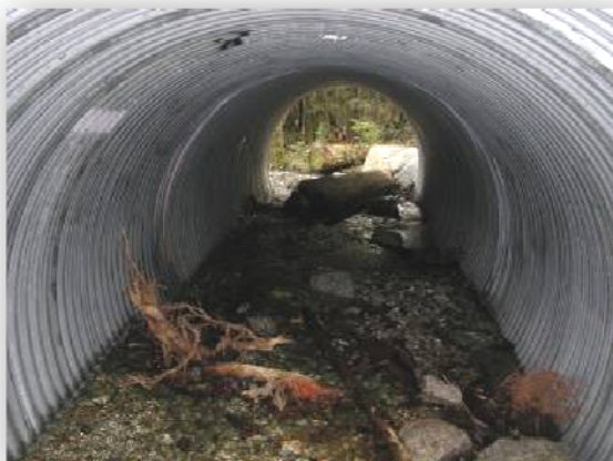
Figures 1a (left) and 1b (right). Looking towards the outlet during 2002 (1a) and 2008 (1b). Despite very heavy rain events since construction, the composition and flat nature of the simulated streambed has not changed significantly over six years; much of the woody debris and boulders are in similar positions.
