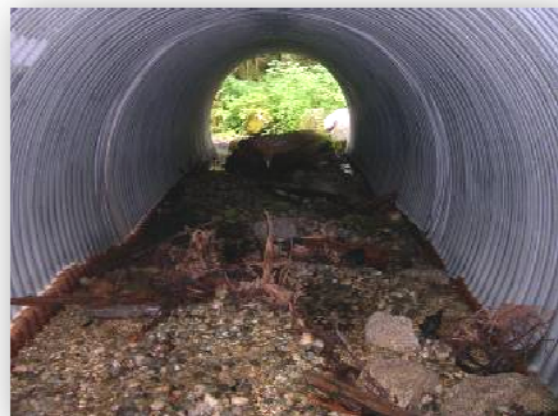
Figures 1a (left) and 1b (right). Looking towards the outlet during 2002 (1a) and 2008 (1b). Despite very heavy rain events since construction, the composition and flat nature of the simulated streambed has not changed significantly over six years; much of the woody debris and boulders are in similar positions.
