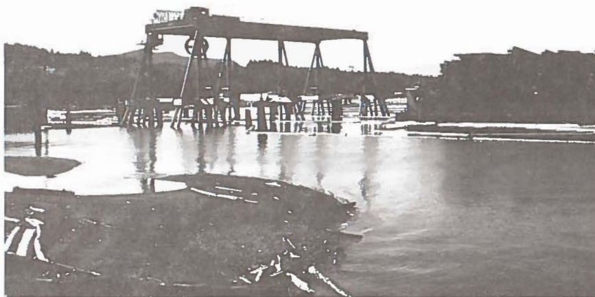
Figure VII-32. Overhead Crane Barge Loader.
