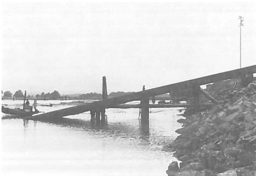
Figure VII-41. Dump Ramp - Steel.
