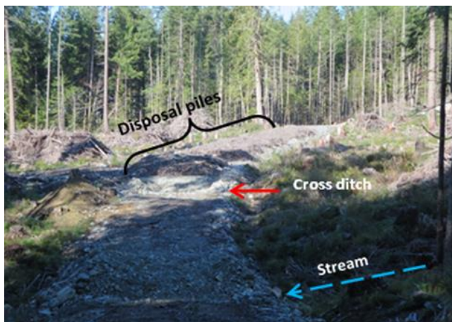
Figure 3. View of stream location at spur 1 and a cross-drain constructed adjacent to a debris pile. A buffer of approximately 45 m was maintained between the disposal pile and the stream.
