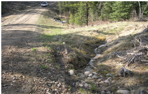
Figure 2. An off-take ditch can be an effective method to evacuate the water away from the road.
