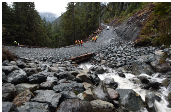
Figure 1. Low water bridges and vented fords allow the passage of high water, large debris and bedload over the structure with a minimum of damage.
