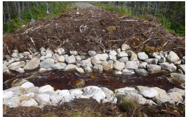
Figure 2. Water crossing structure removal can reduce future maintenance costs and impacts to aquatic habitat related to structure failure.
