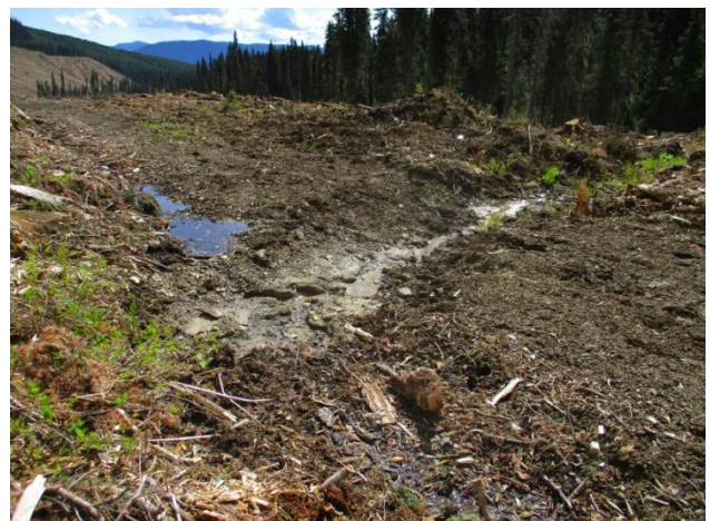
Figure 5. Typical cross-ditch constructed by excavating through frozen soils. Note the sedimentation within the cross-ditch, and the ponded water.
