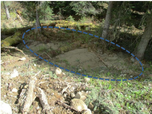
Figure 4. View of the sediment deposition area (dashed oval) immediately downhill from the cross-ditch outlet.
