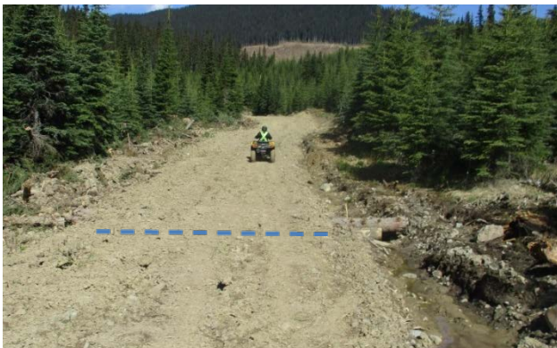
Figure 7. Dashed line indicates location of a log bundle that was left in place during deactivation. The bundle is not passing ditch water that is accumulating uphill of the inlet, and there are signs of sedimentation in the ditch.
