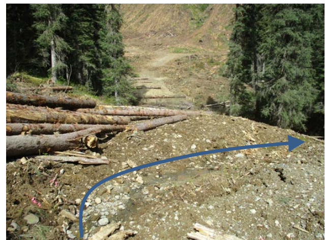
Figure 3. Cross-ditch with water through the flow path and logs left on-site. The arrow indicates the flow path of ditch water entering the cross-ditch.
