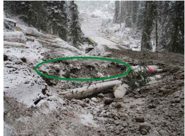
Figure 2. View of inlet of the completed log bundle showing the various log lengths and the position and composition of the ditch block (solid oval).
