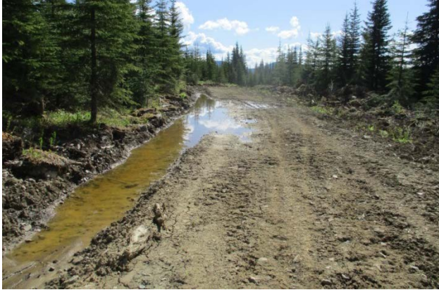
Figure 6. Winter road during spring, showing ponded water along the ditch and road surface. This is a good location to plan for the construction of a cross-ditch.
