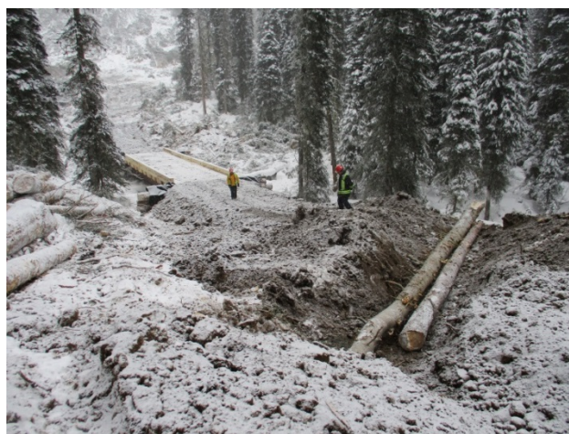
Figure 1. First two logs of a bundle positioned at a skew in the excavation through the road.
