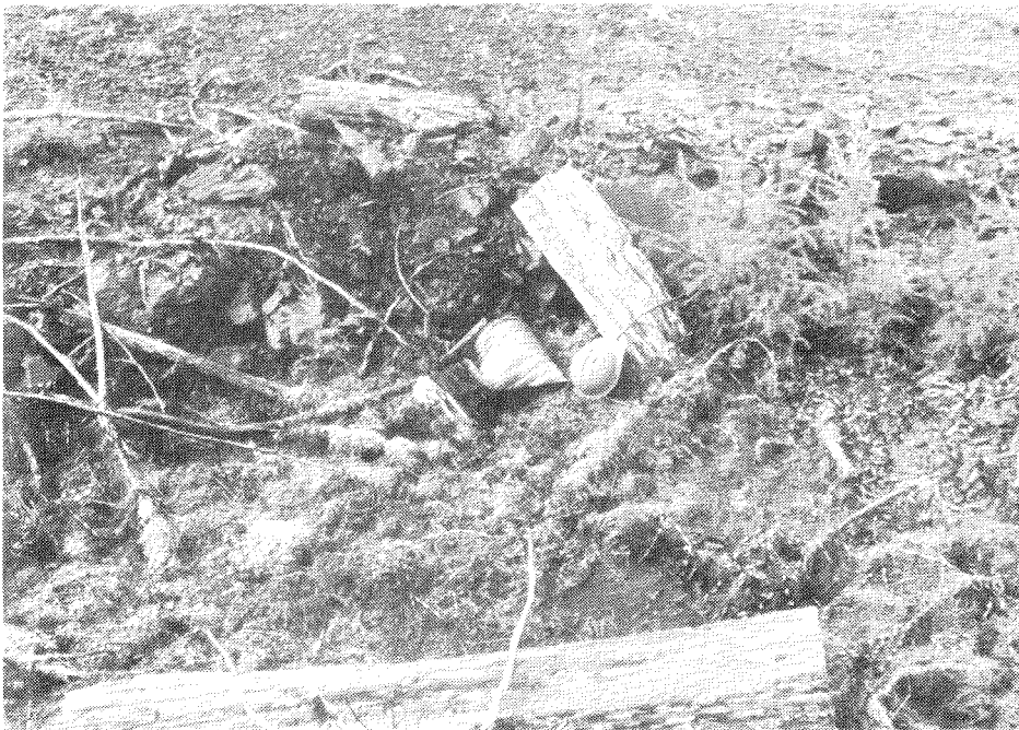
FIGURE A4.3d. Culvert inlet almost plugged with debris and sediment, Example #3.
