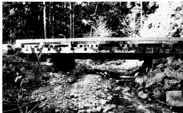
Figure 1. One of the first railcar subframe bridges constructed according to the standard design specifications: built by Wakiwa Construction Ltd. for the BCMOF in 1993.
