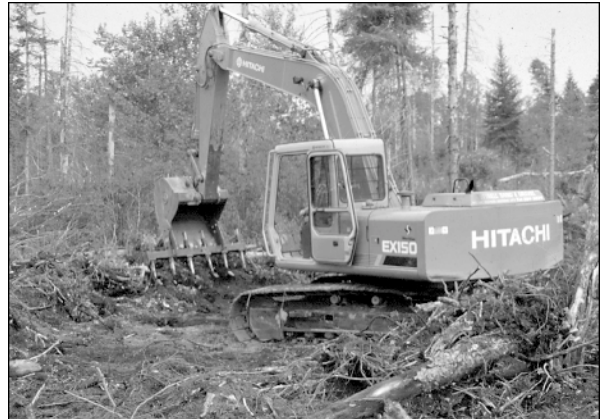
Figure 5. Scalping with a custom-made rake mounted on a Hitachi EX150 excavator.
