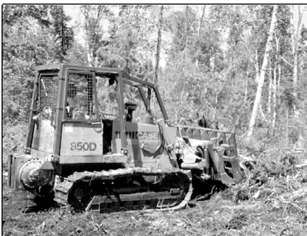
Figure 4. Scalping with a custom-made rake mounted on a Case 850D bulldozer.
