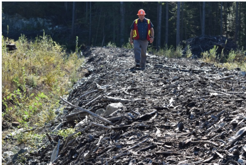
Figure 5. Debris pile on spur 1 illustrates the typical height of 1.2 m, width of 5 m, and shape of the debris piles.
