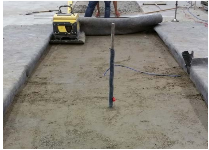
Figure 6. Completed granular base course.
