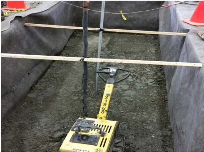
Figure 5. Clay subgrade under construction.
