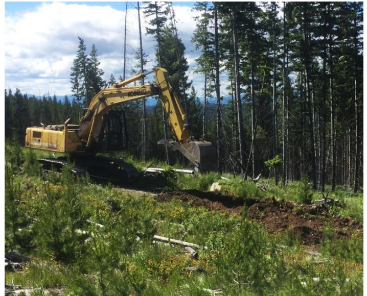
Figure 42. Temporary road rehabilitation and seeding.
