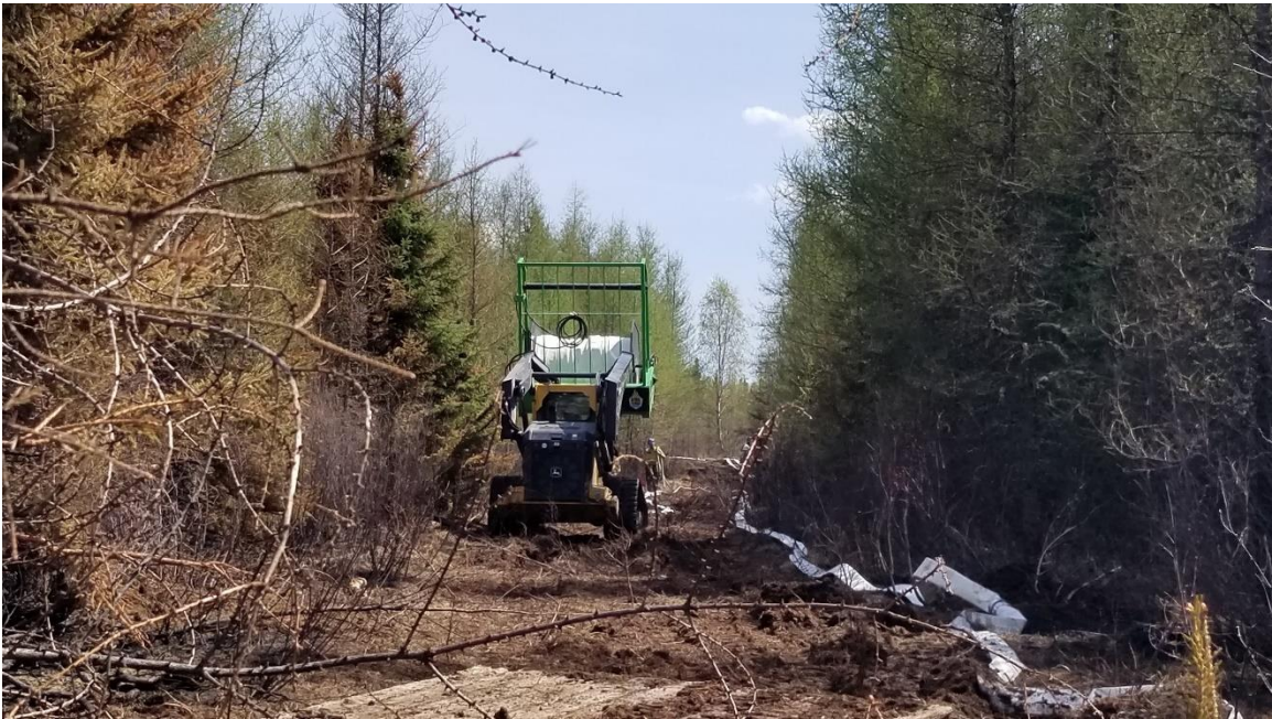
Figure 22. Skid steers moving up and down the cleared path caused the surface to progressively get worse for equipment transport.
