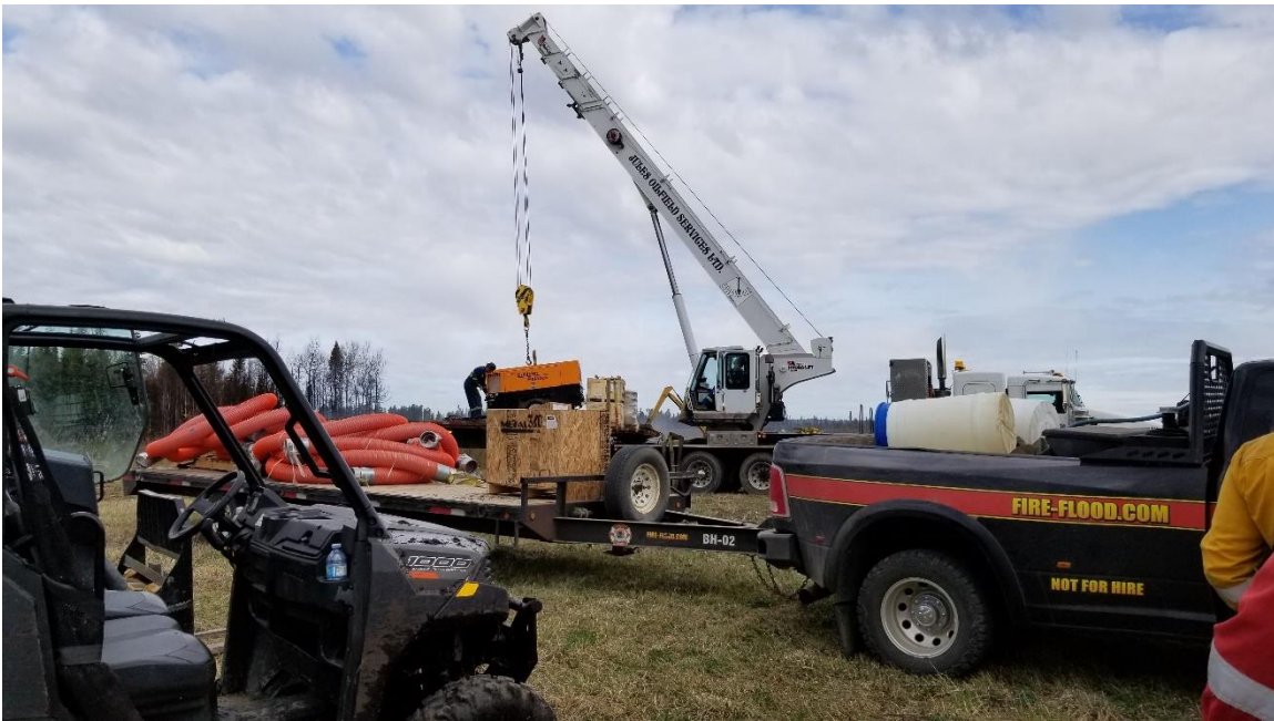
Figure 19. Compressor being off-loaded from the flat-bed. The compressor was not used since temperatures did not fall below fore 0 degrees Celsius.
