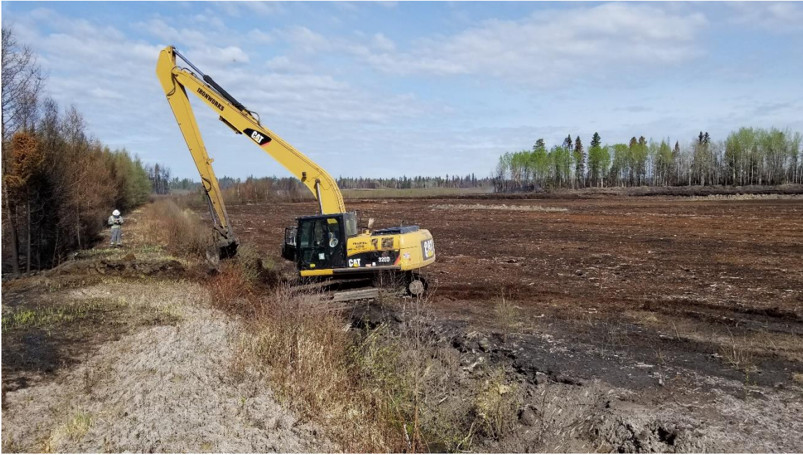
Figure 27. A Parkland County contracted excavator was used to expedite equipment setup. In this instance, the excavator was used to build a dirt bridge.
