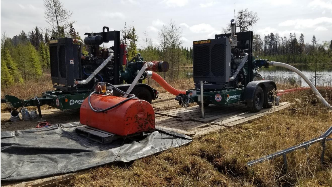
Figure 23. Externally procured rig mats were used to manage wet, soft ground.
