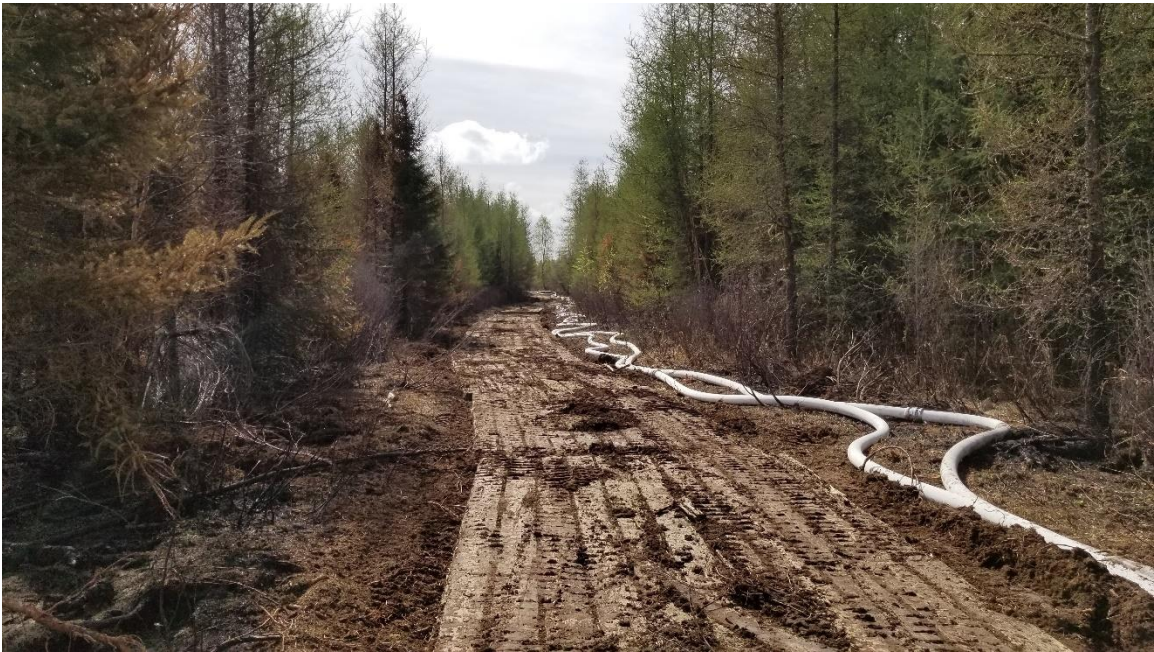
Figure 24. A total of 60 rig mats was used to ensure secure passage from the peat farm to the water source for equipment transport.
