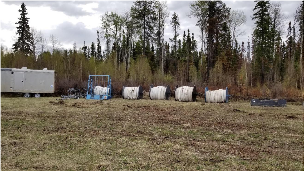
Figure 17. Spools on 4-inch hose, each 0.5 km in length. Total length of 2.5 km.
