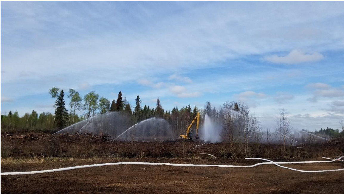
Figure 30. The excavator working in conjunction with the water cannons to put out Hotspot 1.
