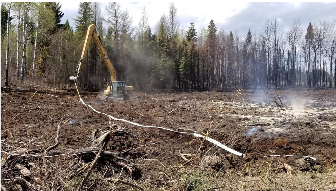
Figure 28. An instance of the excavator assisting in deploying the 4-inch hose around Hotspot 1.
