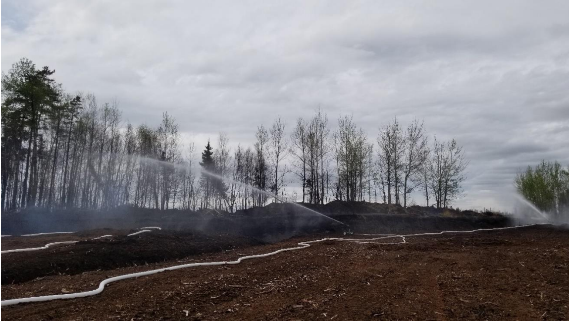
Figure 38. East-bound 4-inch line, 120-meters in length, containing 2 water cannons.
