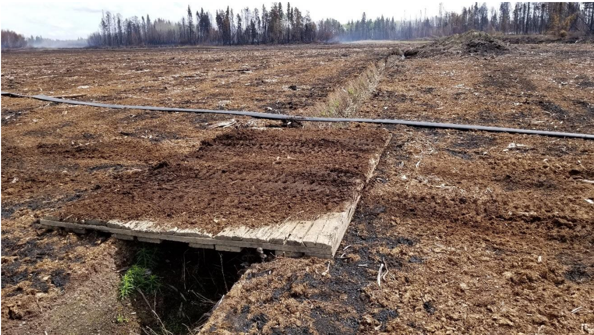
Figure 26. Rig mats used as a temporary bridge across drainage channels.
