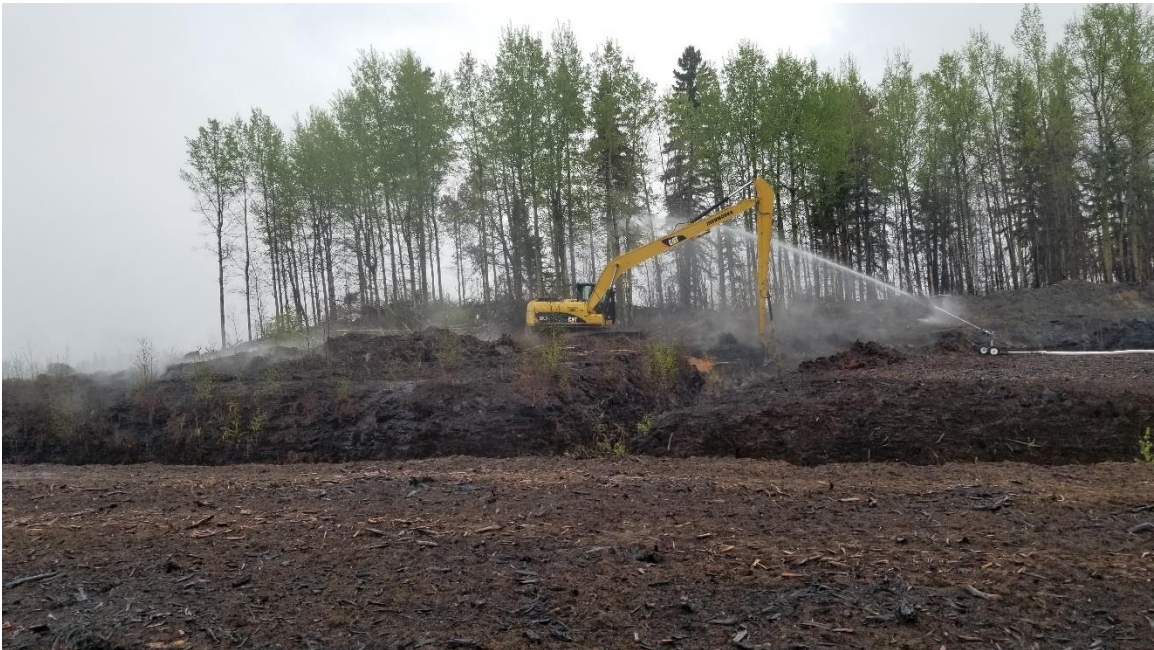
Figure 41. The excavator checking for hotspots beneath the surface where water cannon operations occurred on Hotspot 3.
