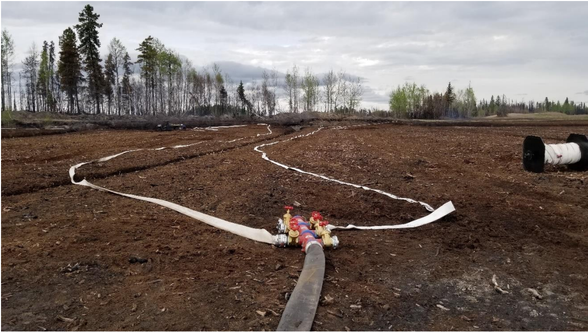
Figure 34. Manifold reducing 6-inch line main line (black hose) to 4-inch off-shoots (white hose).
