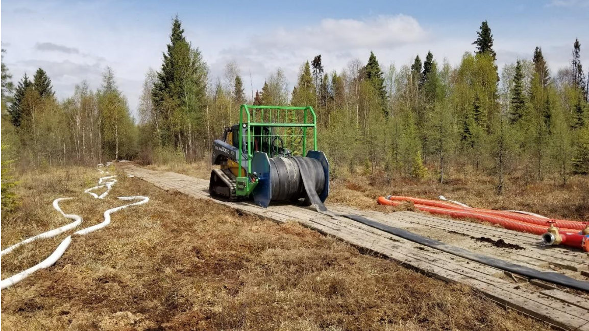
Figure 33. 6-inch hose being unspooled on rig mats.
