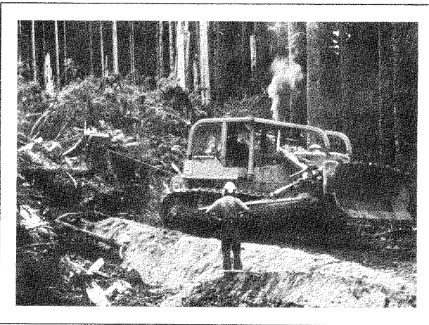
Figure 2-c. Bulldozer removes an anchor stump
