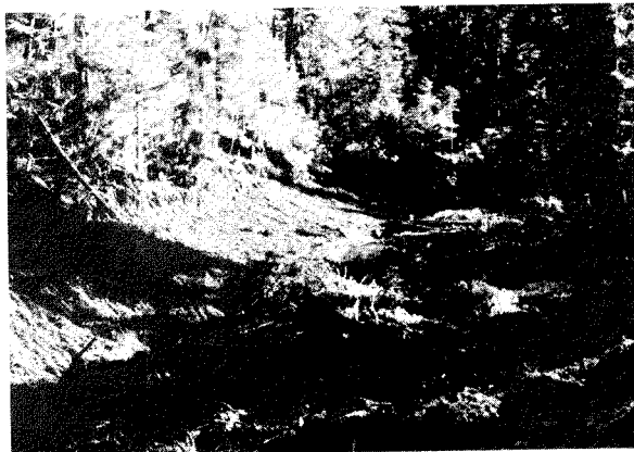
Figure 1-b. Waste material to be covered with subsoil to form the subgrade
