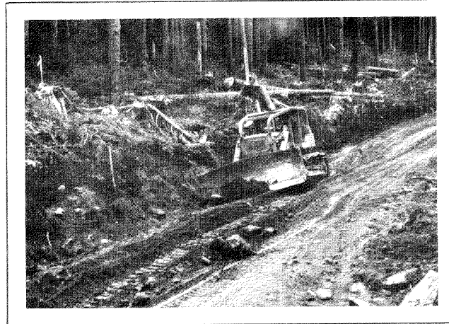
Figure 2-e. Bulldozer prepares ditch.
