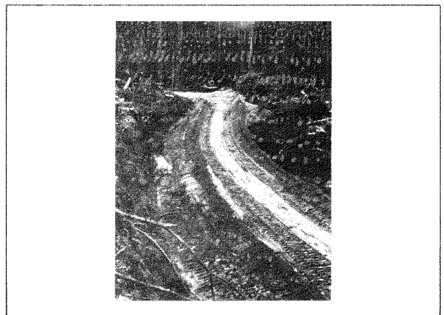
Figure 2-g. Mineral soil was used to finish the subgrade.
