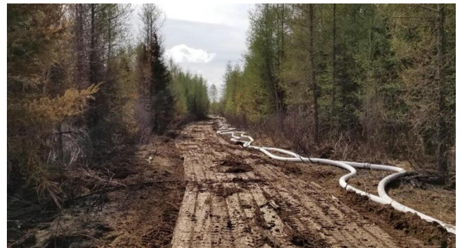
Figure 1. Tracked skid steers damaged soft ground. Rig mats were required thereafter.
