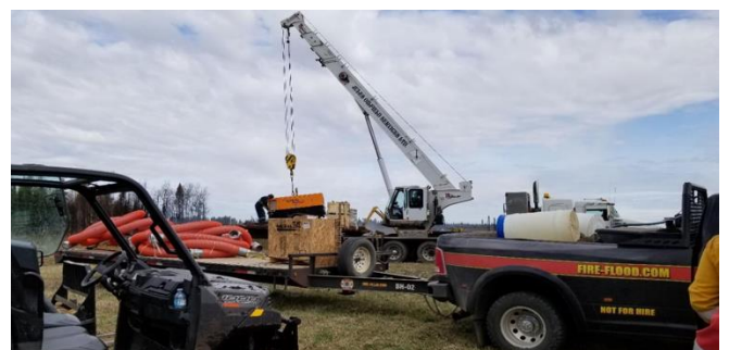
Figure 3. Large staging area required for equipment.
