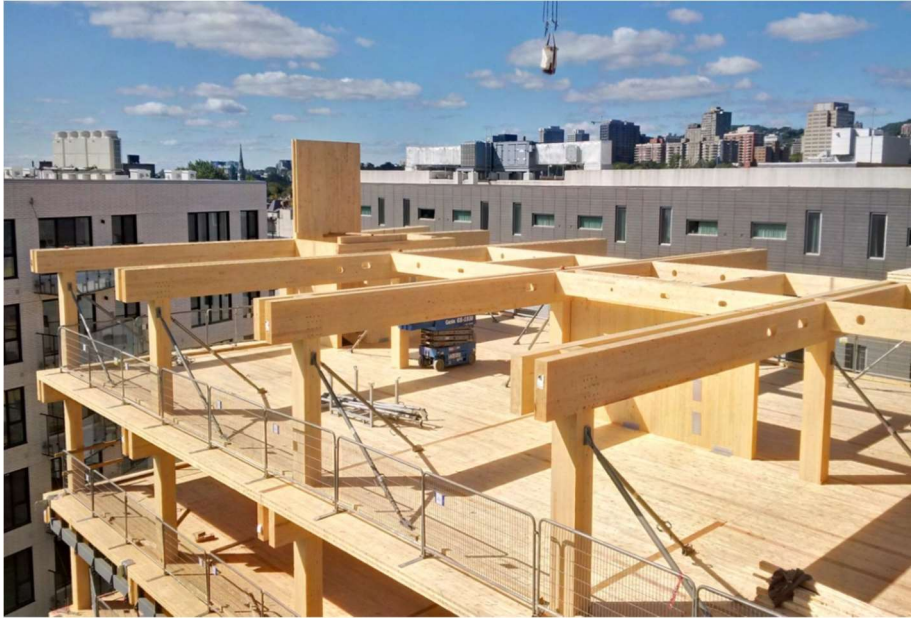
Figure 2. CLT floors on supporting beams in a post-and-beam construction
