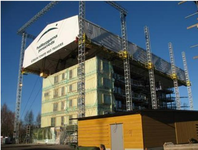
Figure 5. Using a liftable temporary roof to protect timber construction in Sweden.
