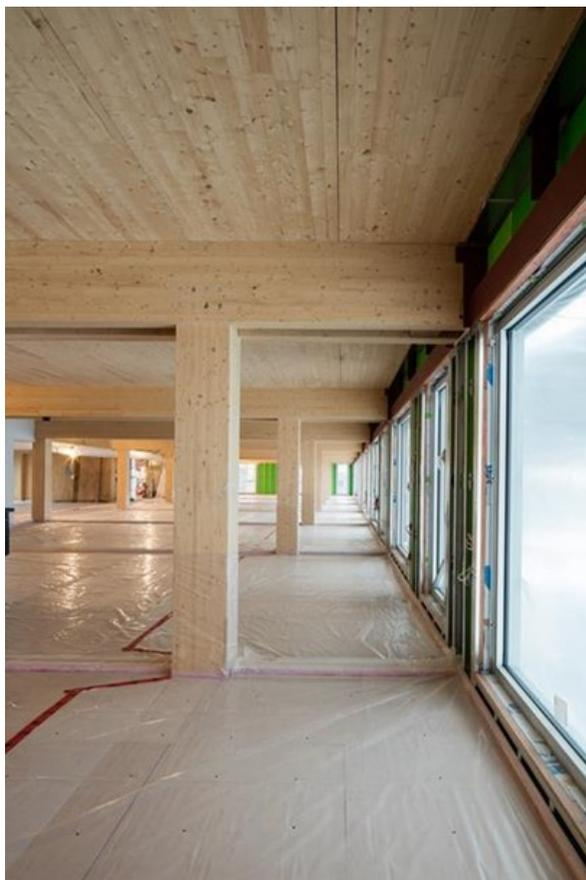
Figure 4. A floor is made watertight using plastic sheets in a mass timber building in Montreal.
