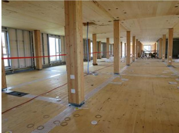
Figure 3. Joints between CLT floor panels sealed with tapes in a project in Vancouver.
