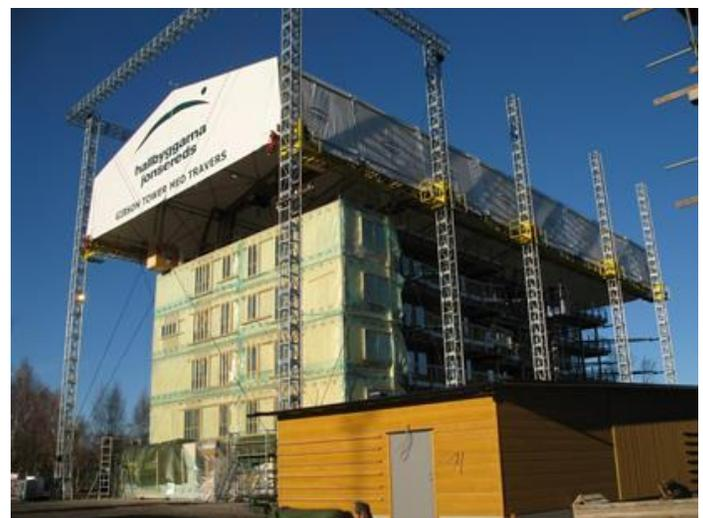
Figure 7. Using a liftable temporary roof to protect timber construction in Sweden.
