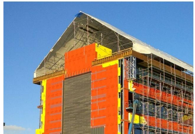
Figure 6. Using a temporary tent to protect roof construction in a Vancouver project (photo credit: RDH Building Science).
